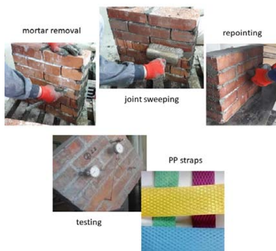
Figure 1. Structural repointing and testing in STREP
