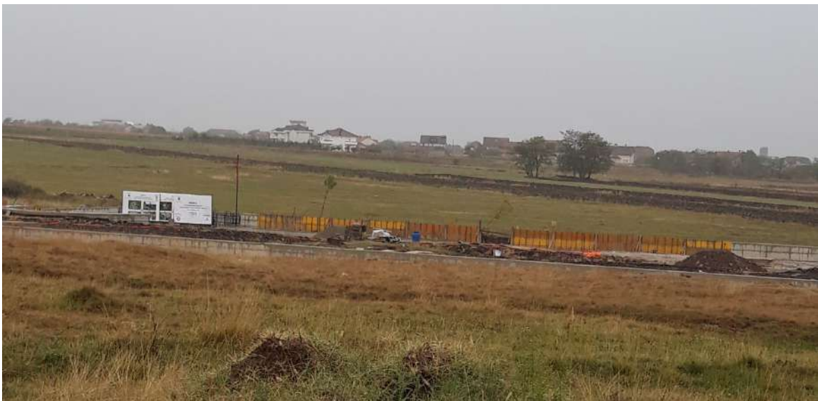
New construction (ID 17).
